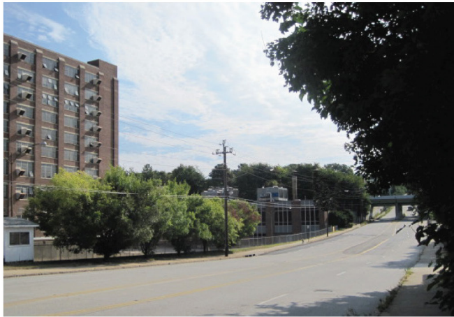
NORTH AVE./BELTINE, EXISTING CONDITION
